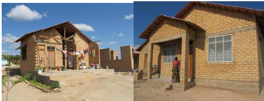
Picture 5 - Houses are built incrementally, allowing the new owner to move in when half built and then gradually complete the construction
